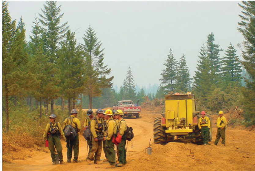
Roads that divided inventoried roadless areas were widened and improved in preparation for burnout operations on the Biscuit Fire.
